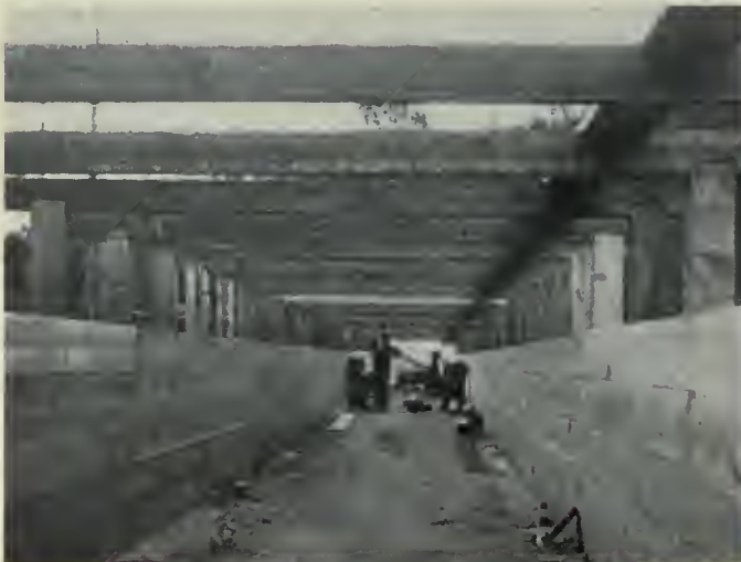
Fig. 4—Flume System, Hydro Plant—Kamloops, B. C.
